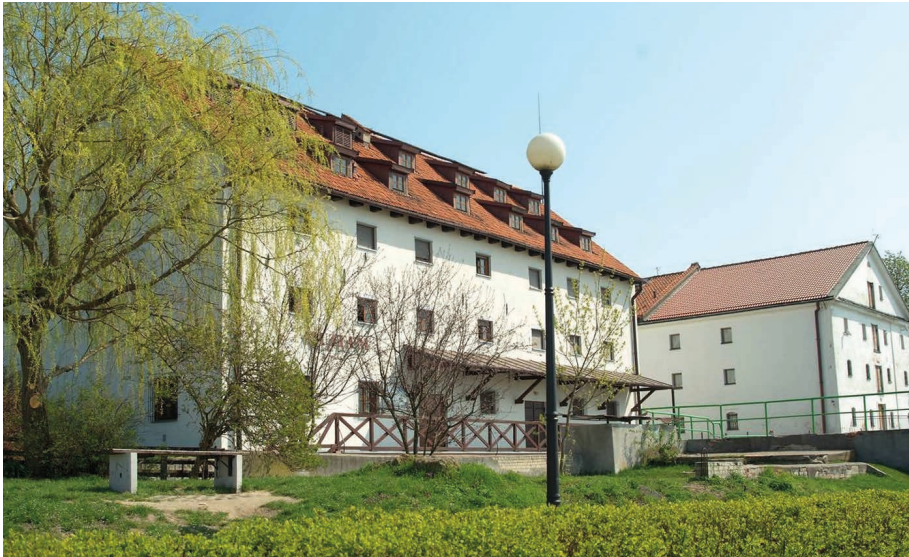
Fig. 19. The historic granary at 11b Kazimierz Wielki Street – the seat of the Department of Ethnography, the place of presentation of two permanent exhibitions: The Culture of Masovia in the Folk Vision of the World and The Art of the Far East. Płock's Treasures of Buddhist Asia
